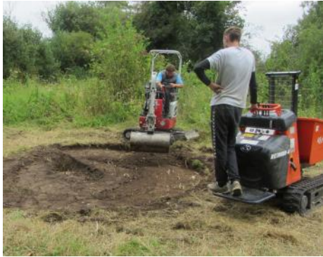
The new pond being dug at Millhoppers
